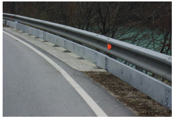
Fig. 9. Guardrail with additional protection for PTW riders: application on road section.
